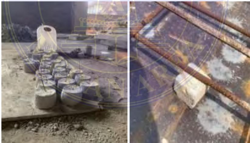
Gambar 3.40 Beton Decking
