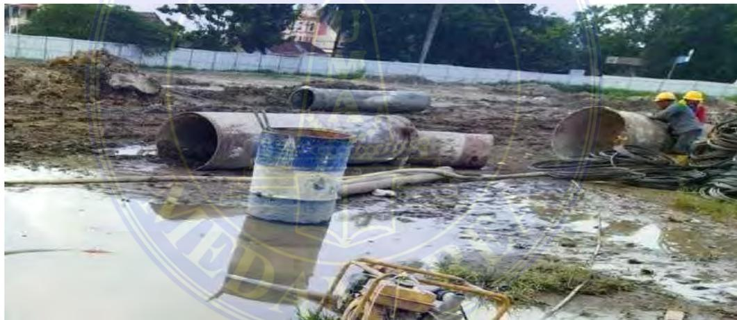
Gambar 14. *Casing bored pile*
