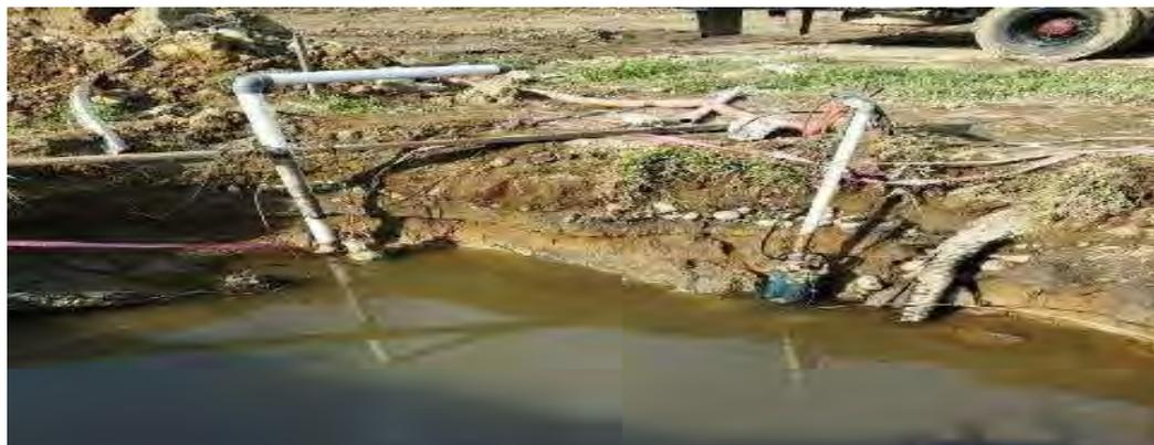
Gambar 21. Pompa Submersible
