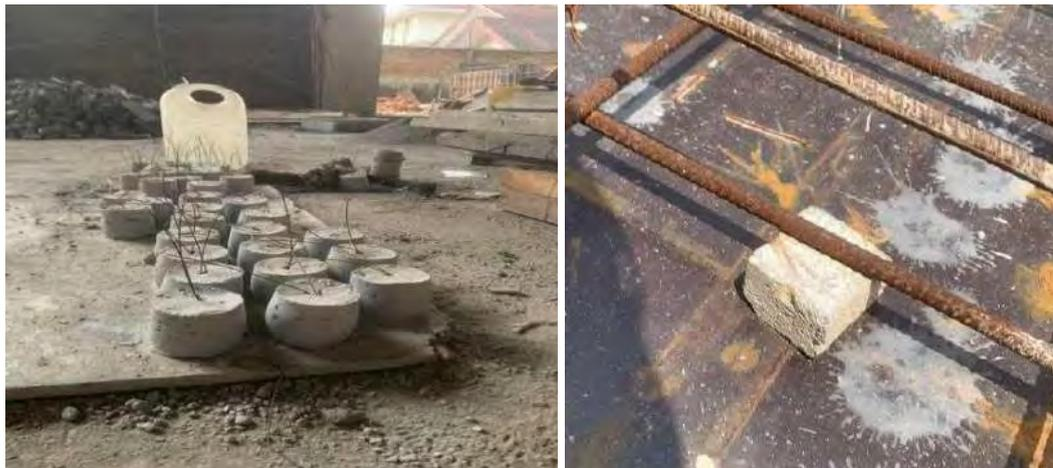
Gambar 40. Beton Decking
