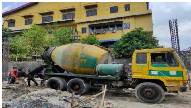
Gambar 3.5 Truck Mixer beton
