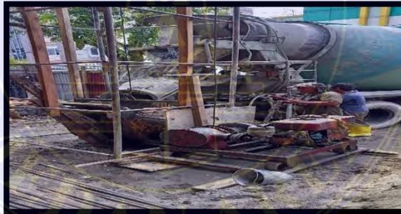
Gambar 3.1 17 Lift Cor Beton
