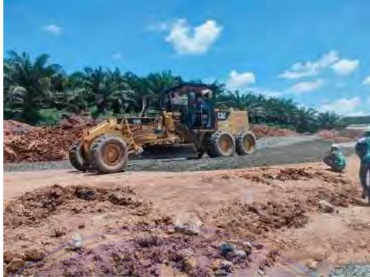
Gambar 3.1.25 Motor Grader
