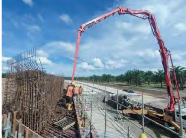
Gambar 3.1.14 Pompa Beton/*Concrete Pump Truck*
