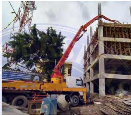
Gambar 3.2 *Concrete Pump*
