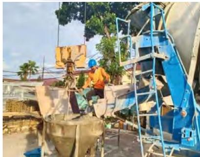
Gambar 3.3 *Concrete Bucket*
