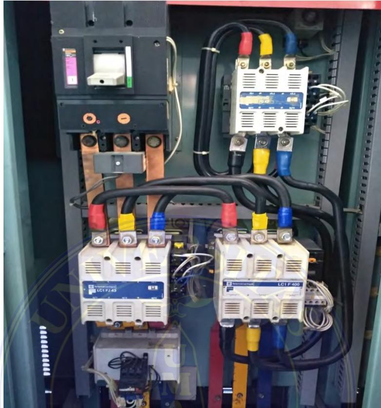
Gambar 9 Panel Kontrol *Starting* Motor Dengan Metode *Start Delta*
