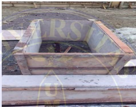
Gambar 4.10 Bekisting Pile Cap
