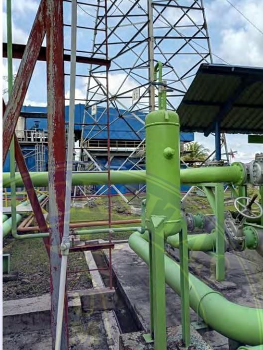
Gambar 3.1 Tanki Pengecekan Level Air Demin Di Tanki Reservoir
