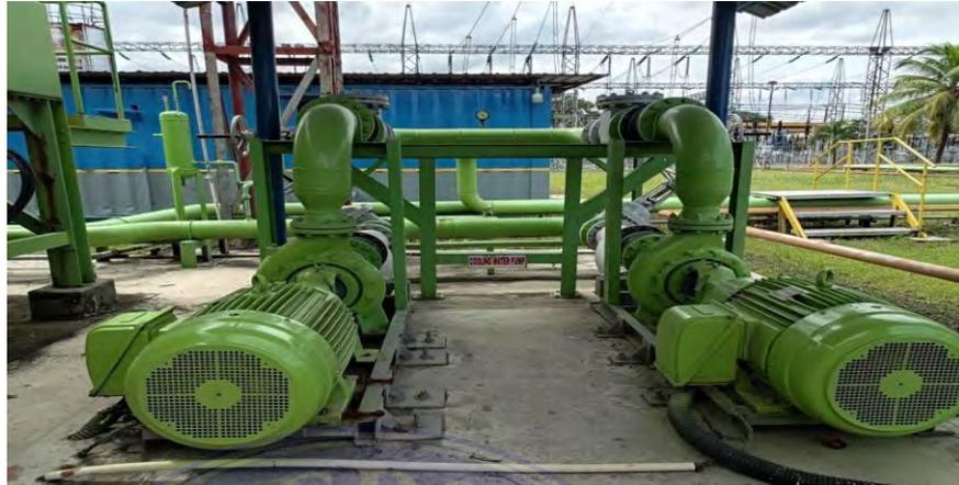
Gambar 3.5 Cooling water pump
