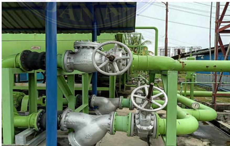
Gambar 3.2 Valve In Cooling Water Pump
