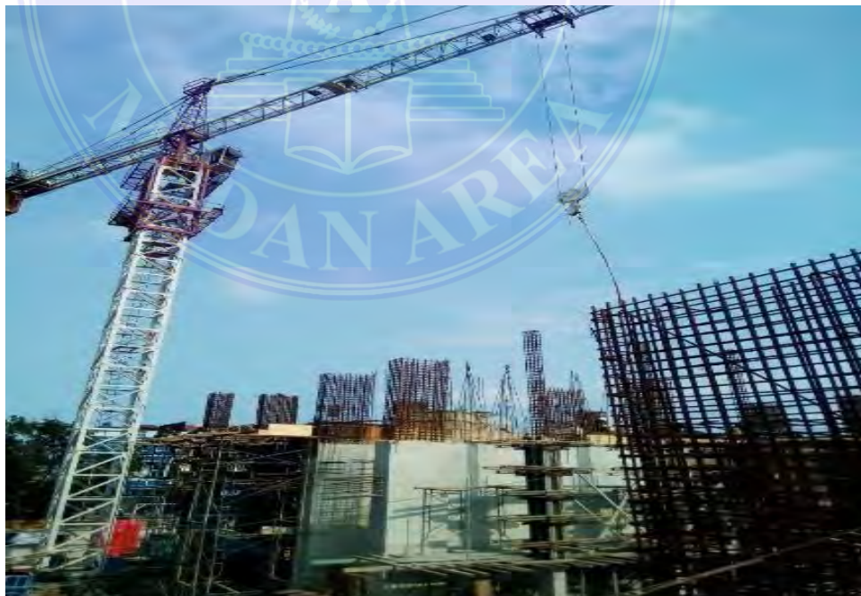
Gambar 3.5 Tower Crane (TC)
