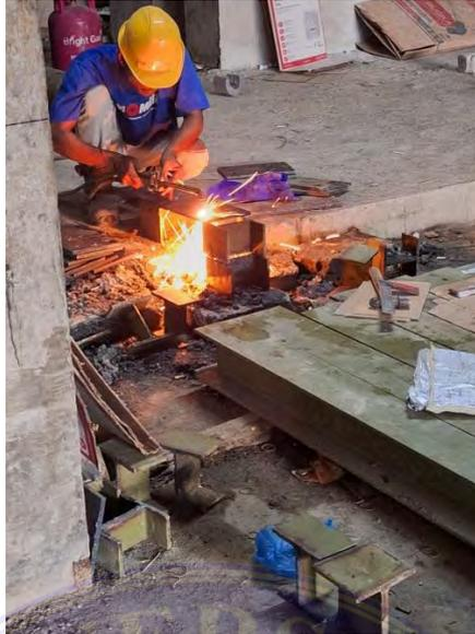
Gambar 4.3 Pemotongan *H-Beam*
