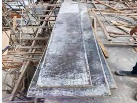
Gambar 3.1.7 Bekisting (Kolom)
