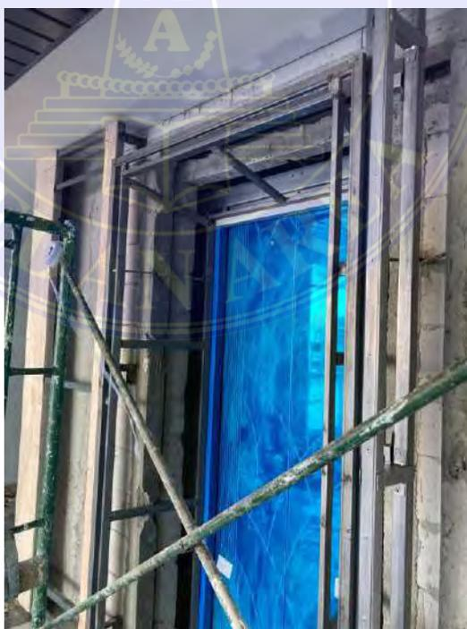
Gambar 3. 13 : Pemasangan Rangka besi hollow openingan lift lantai 3-7
