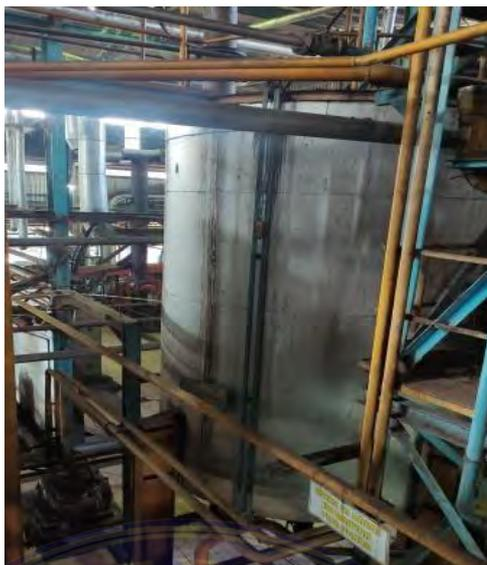
**Gambar 3. 39 Sludge Tank**
