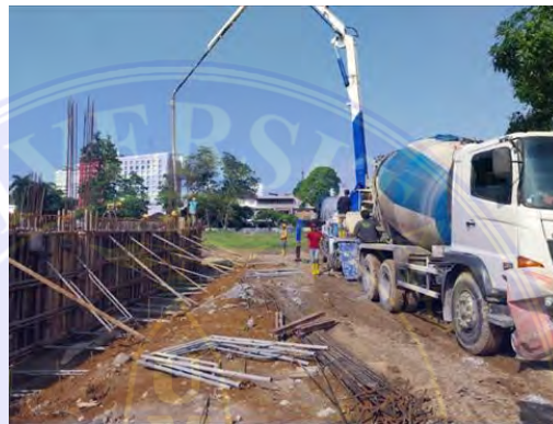
Gambar 3.14 Concrete Pump
