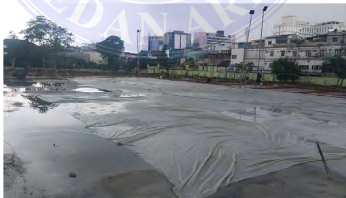
Gambar 4.6 Proses curing
