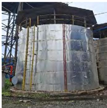
**Gambar 3.39 Feed Water Tank**
