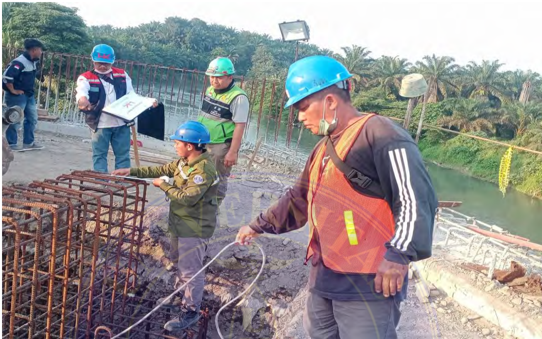
Gambar 1. Pengecoran Balancing Beam
