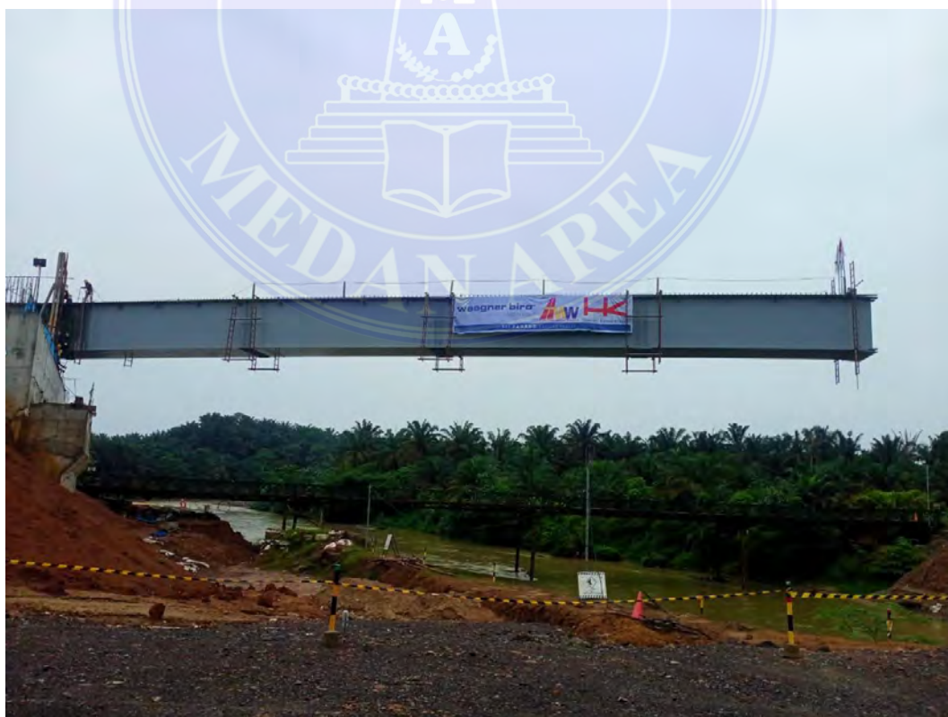
Gambar 6. Erection steel box girder
