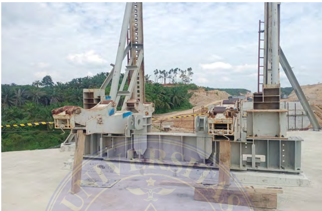
Gambar 3. Perakitan Lower Tower Erection
