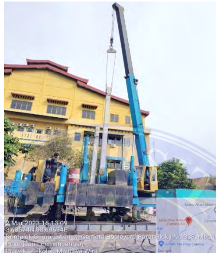
Gambar 3.31 Hydraulic static pile driver Sumber : Dokumen Lapangan
