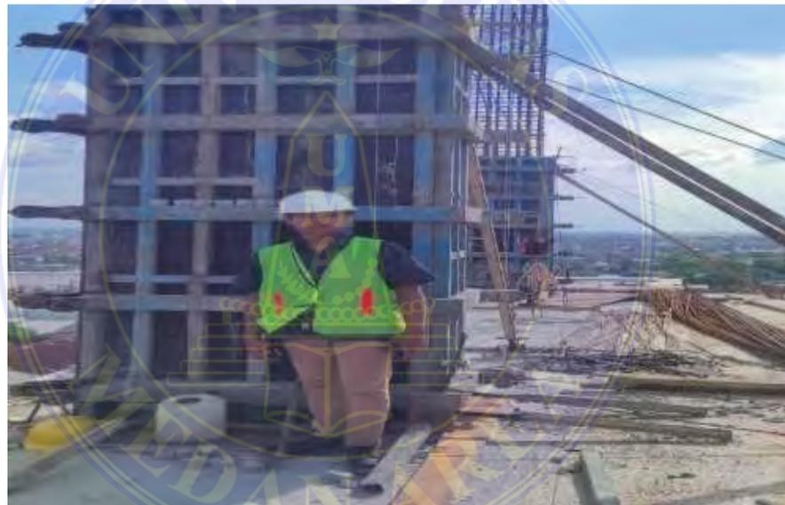
Gambar .4 .Peninjauan bekisting kolom
