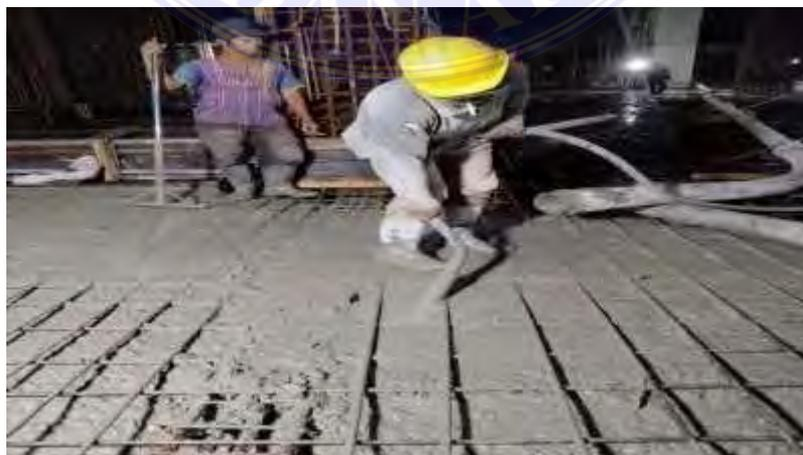
Gambar 3. 12 Concrate Vibratrion
