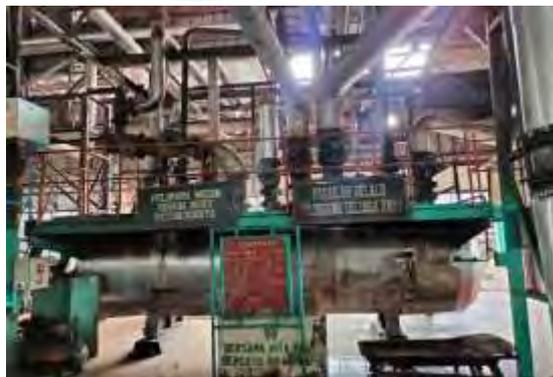
**Gambar 3. 28 Back Pressure Vessel (B.V.P)**
