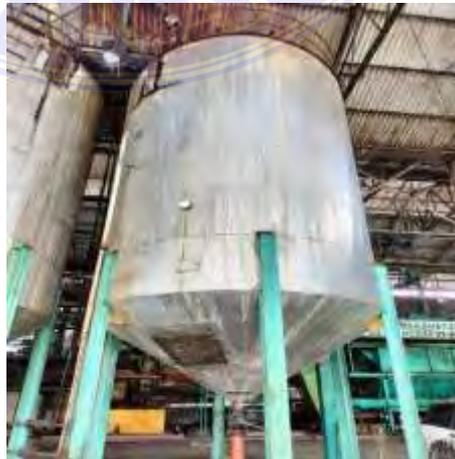
**Gambar 3. 7 Clarifier Settling Tank (CST)**
