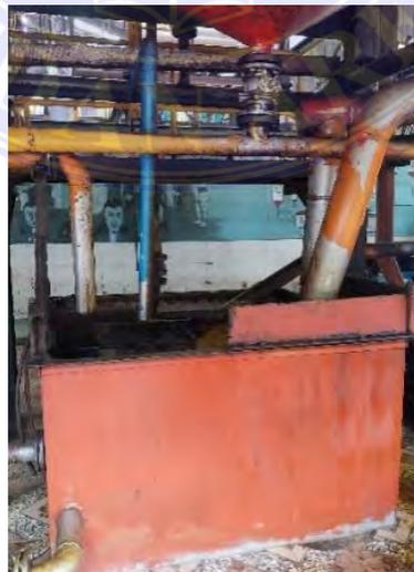
Gambar 3. 34 Sludge drain tank
