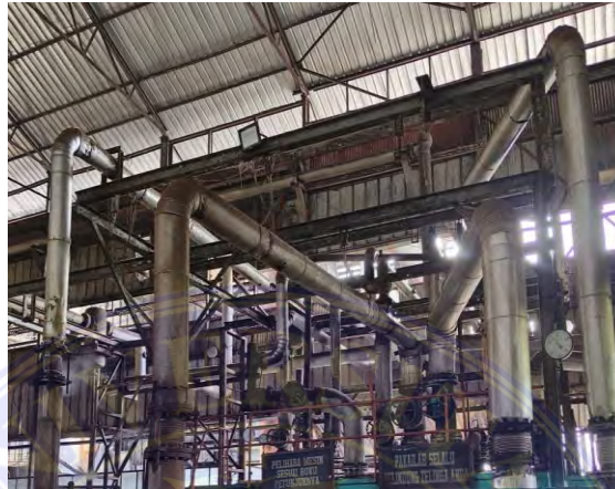
Gambar 3. 60 Back Pressure Vessel (BPV)
