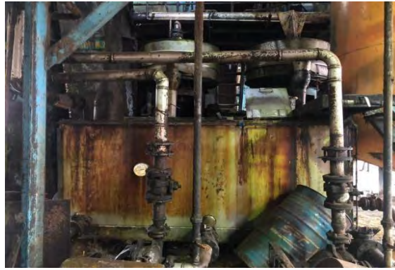
Gambar 3. 37 Crude Oil Tank
