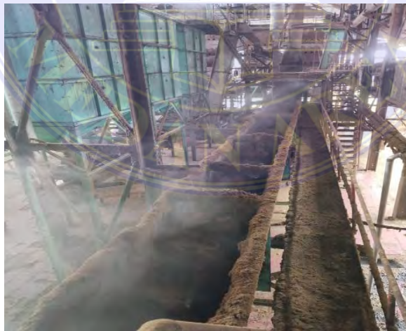
Gambar 3. 44 Cake Breaker Conveyor (CBC)
