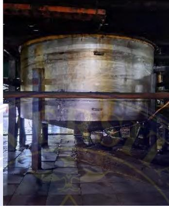
Gambar 3.15. *Sand Trap Tank*
