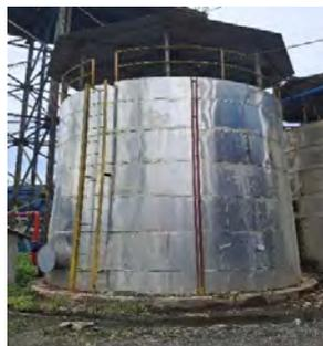
Gambar 3.39. *Feed Water Tank*
