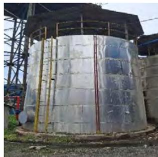
**Gambar 3.39 Feed Water Tank**
