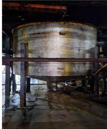
**Gambar 3.15 Sand Trap Tank**
