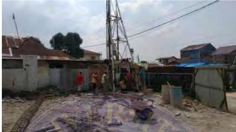
Gambar 4. 7 Pengecoran Bore Pile
