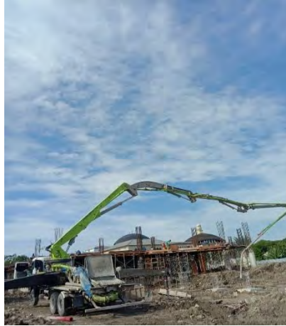
Gambar 2.16 Concrete Pump Sumber: Data Lapangan 2023
