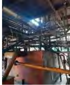
Gambar 3. 19 Crude Oil Tank
