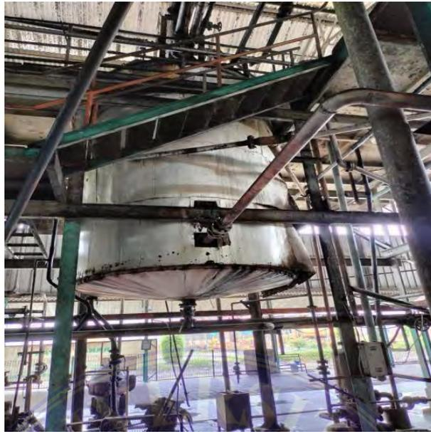
**Gambar 3. 12. Sludge Tank**
