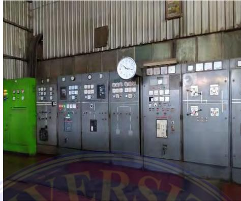
Gambar 3.57 Main Switch Distribution Board ( Panel Kontrol Utama )
