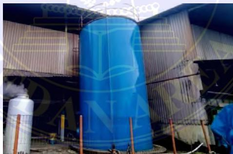
Gambar 3.64 Feed Water Tank
