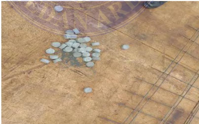
Gambar 3.40 Beton *Decking*
