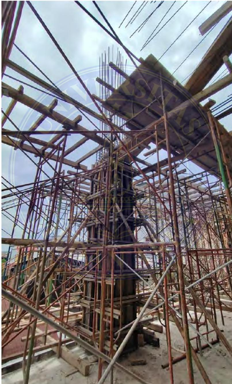
Gambar 4.4 Bekisting Kolom
