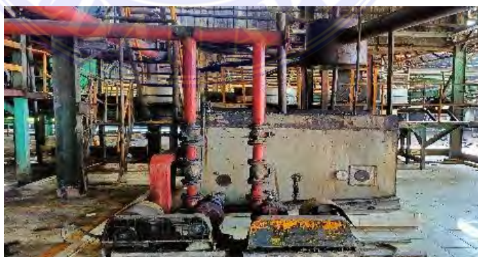
Gambar 3.43 Light Phase Tank
