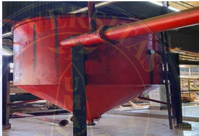
Gambar 3.32 Sand Trap Tank
