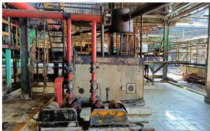
Gambar 3.34 Crude Oil Tank
