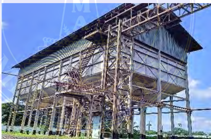
Gambar 3.31 KSB (Kernel Silo Bin)
