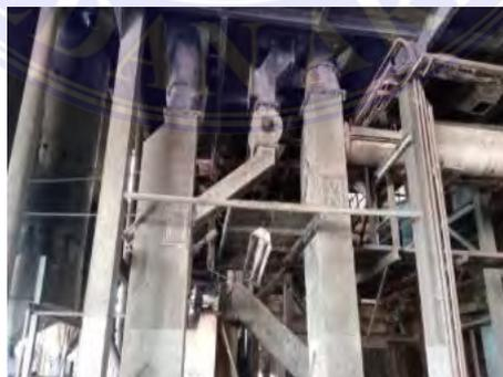
**Gambar 3.26 Light Tenera Dust Separation (LTDS 1 LTDS 2)**
