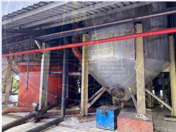
Gambar 3. 14 Continuous Settling Tank (CST)
