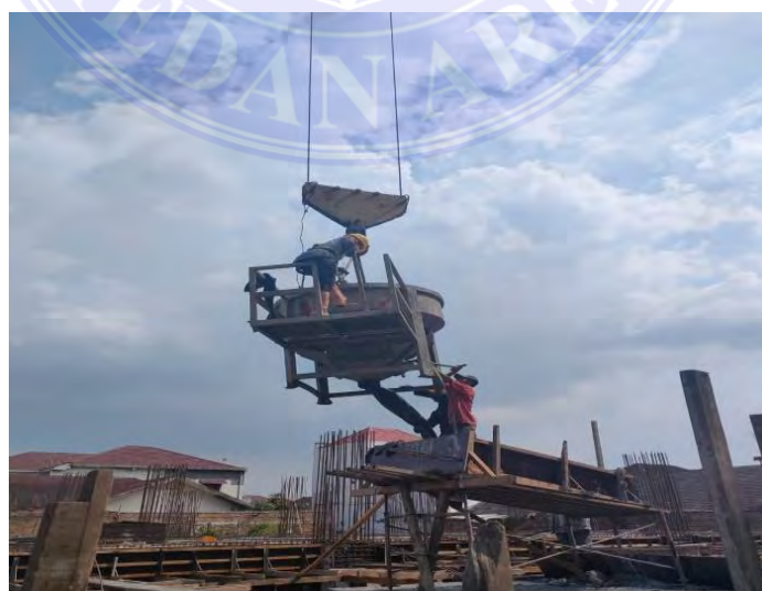
Gambar 3.12 Beton Ready Mix
