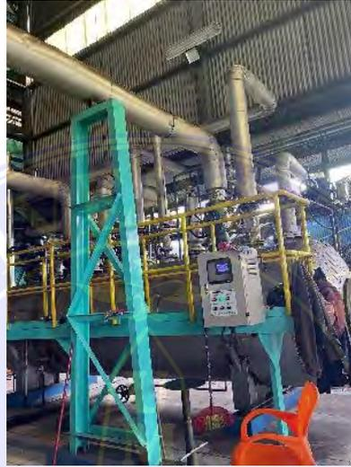
**Gambar 3. 31 Back Pressure Vessel**
