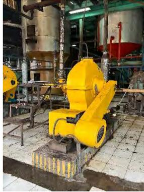
**Gambar 3. 16 Sentrifuse Minyak (*Oil Purifier*)**
