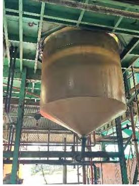
**Gambar 3. 15 Sludge Tank**
