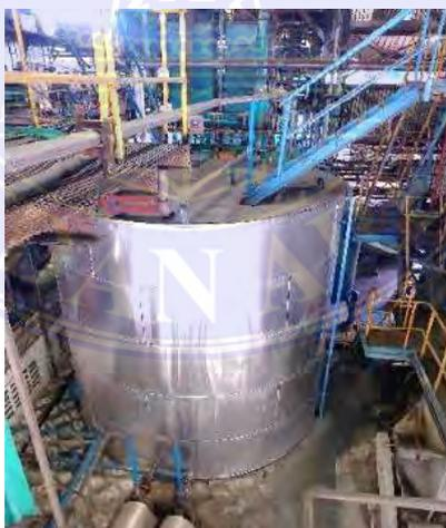
**Gambar 3. 55** *Feed Water Tank*
