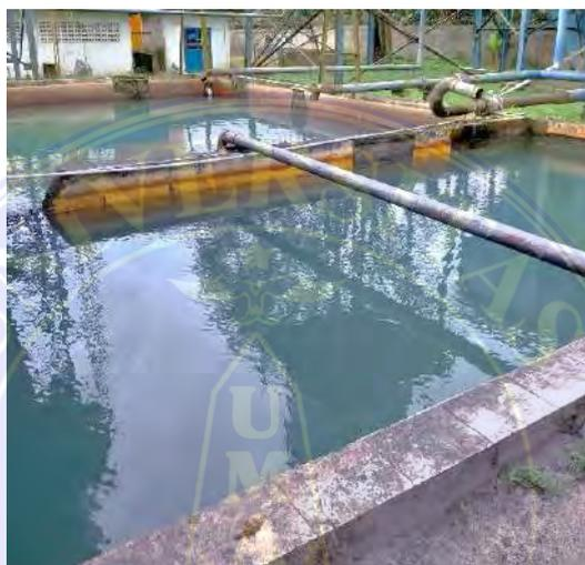
Gambar 3. 50 Bak Sedimen
