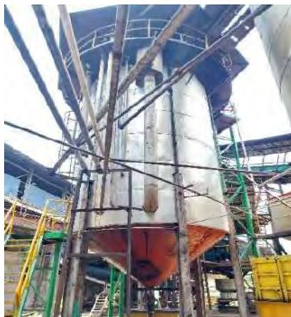
**Gambar 3. 24** *Vertical Clarifier Tank*
