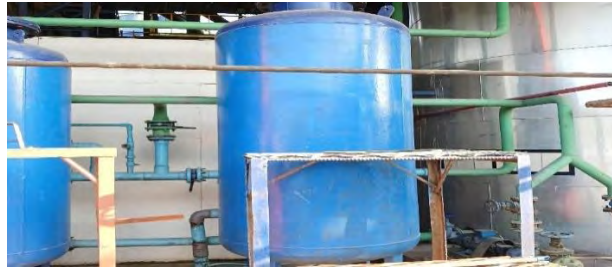
Gambar 3. 38 Carbon Filter
