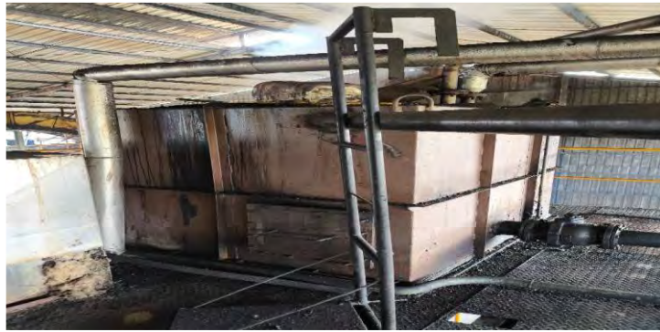
Gambar 3. 13 Buffer Tank
