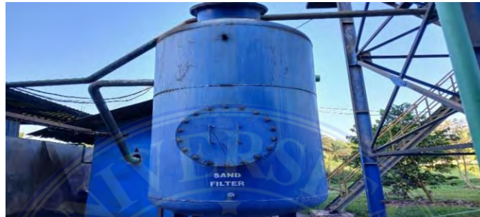
Gambar 3. 37 Sand Filter
