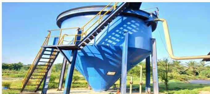
Gambar 3. 35 Clarifier Tank
