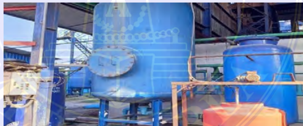
Gambar 3. 39 Softener Tank
