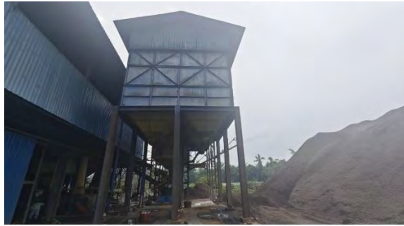
Gambar 3. 30 Kernel Bunker
