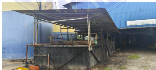
Gambar 3. 20 Recovery Tank
