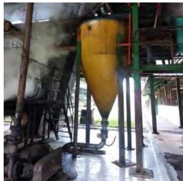
**Gambar 3. 30 *Sand Trap Tank***
