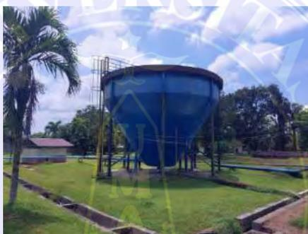
**Gambar 3. 81 Water Clarifier Tank**
