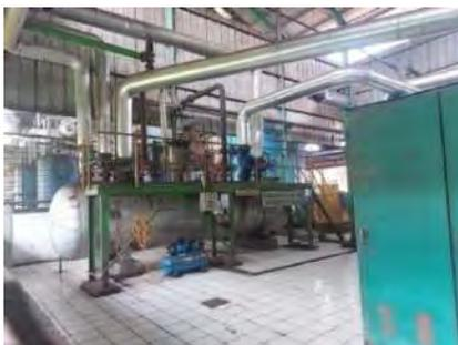
**Gambar 3. 77 Back Pressure Vessel**
