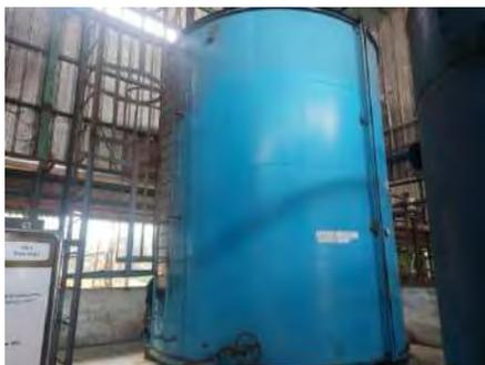
**Gambar 3. 91 Boiler feed water tank**
