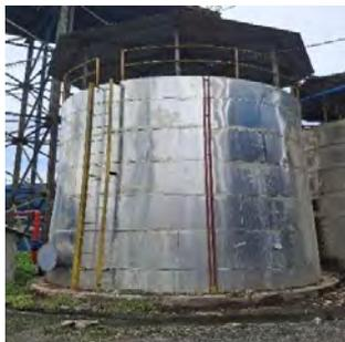
**Gambar 3. 41 Feed Water Tank**
