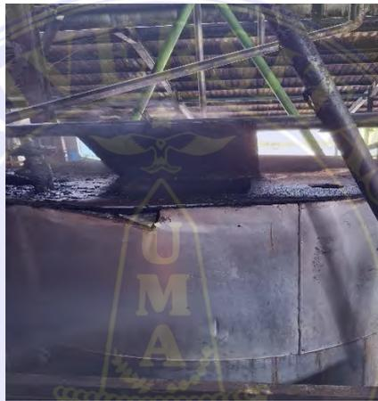
**Gambar 3. 22 Sludge Tank**
