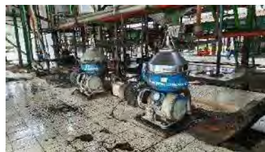
Gambar 3. 38. Sludge Separator
