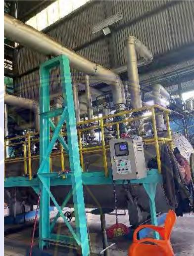
**Gambar 3. 31 *Back Pressure Vessel***
