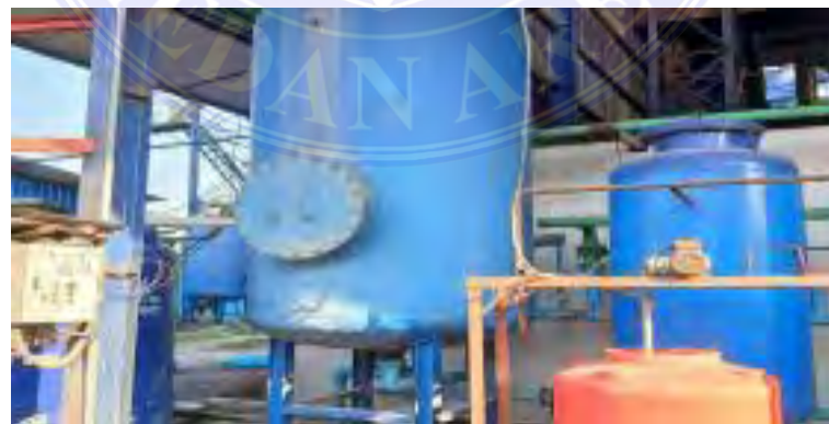
Gambar 3. 40 Softener Tank
