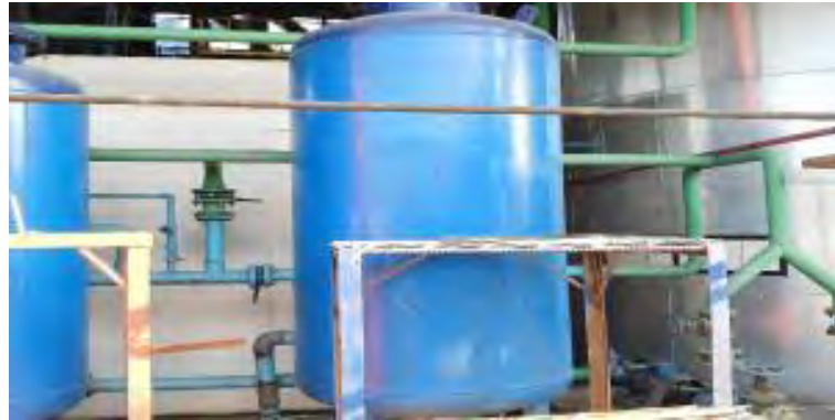
Gambar 3. 39 Carbon Filter
