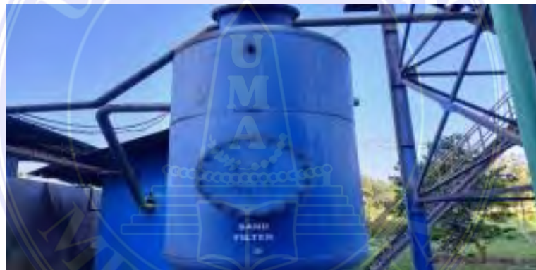
Gambar 3. 38 Sand Filter
