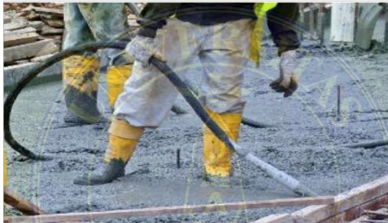
Gambar 13 Concrete Vibrator
