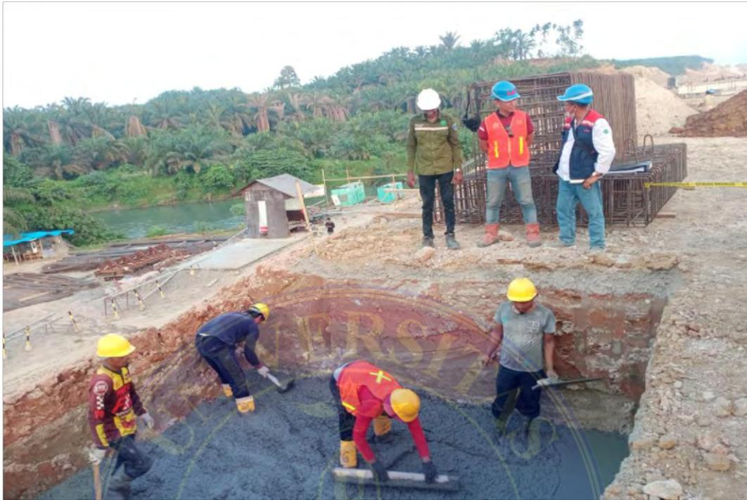
Gambar 38 pengecoran Balancing beam
