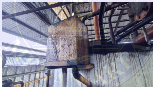
Gambar 3. 30 Float Tank
