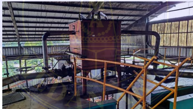
Gambar 3. 26 Distributor Tank
