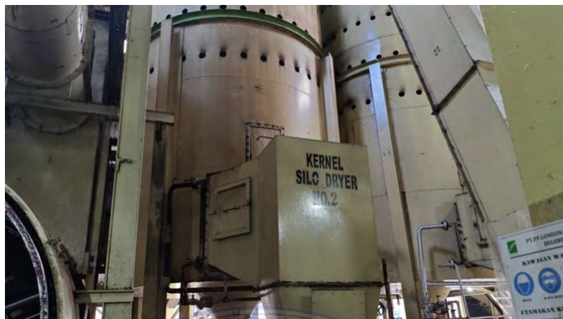
Gambar 3. 52 Kernel Silo Dryer
