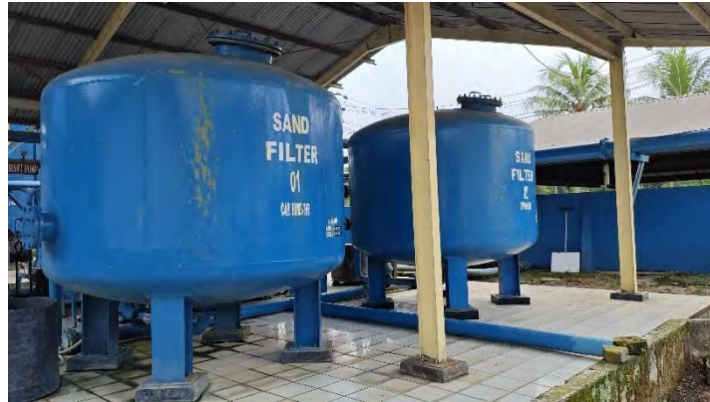
Gambar 3. 58 Sand Filter
