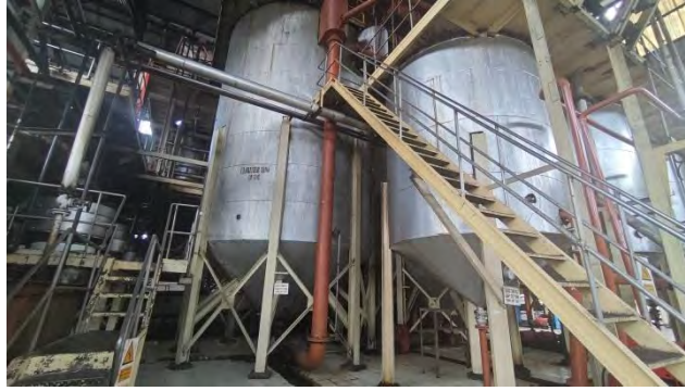
Gambar 3. 27 Clarifier Tank
