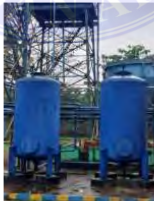
Gambar 3. 46 Sand Filter
