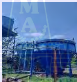
Gambar 3. 44 Clarifier Tank
