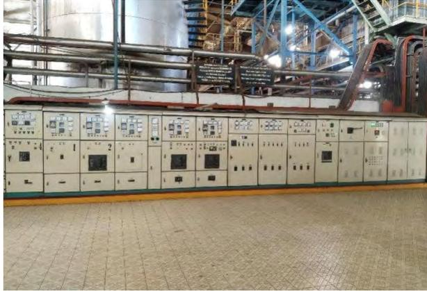
**Gambar 3.68 Panel – Panel Listrik ( Main Switch Boarf )**
