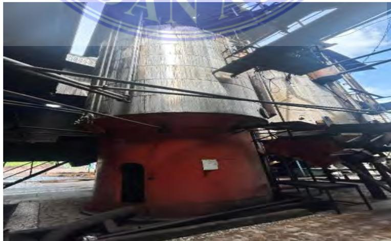
**Gambar 3. 36 Vertical Continuous Tank**
