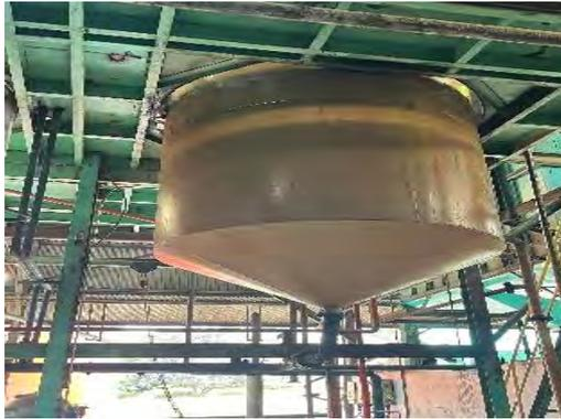
**Gambar 3. 15 Sludge Tank**
