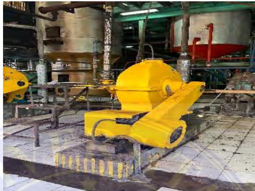
**Gambar 3. 16 Sentrifuse Minyak (Oil Purifier)**
