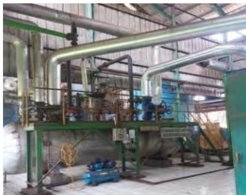
Gambar 3. 85 Back Pressure Vessel
