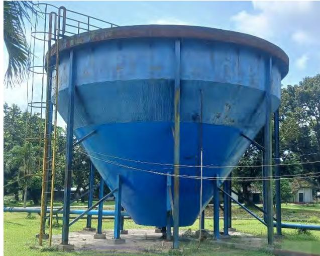
**Gambar 3. 76 Water Clarifier Tank**
