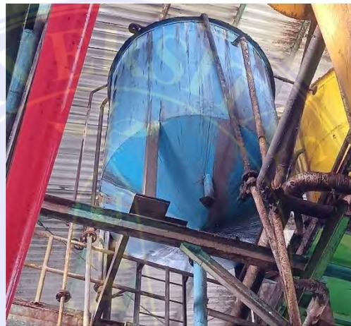
Gambar 3. 45 *Water Dilution Tank*
