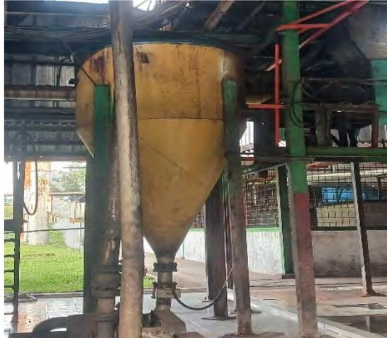
**Gambar 3. 27 Sand Trap Tank**
