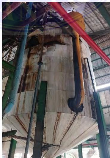
**Gambar 3. 31 Continuous Settling Tank**
