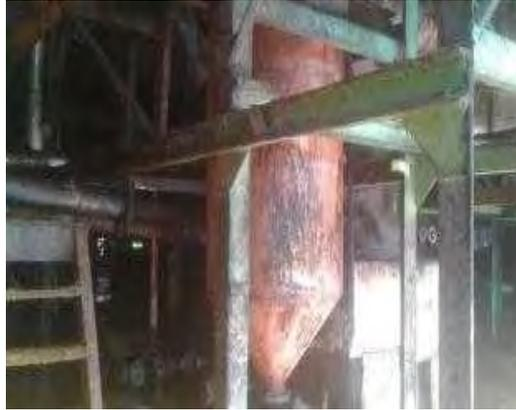
Gambar 3. 29 Sand Trap Tank
